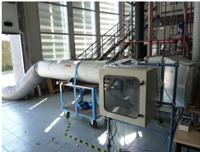
Figure 6: Wind tunnel exhaust.
