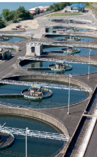
A modern wastewater treatment plant
