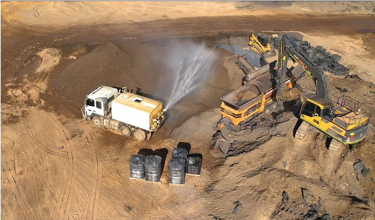
**Figure 18** In-Situ Application of S/S for PFAS Treatment (McDonough et al., 2021)
