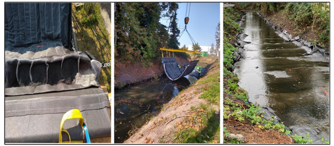
Figure 3: Construction of reactive mat in the Lieve.
