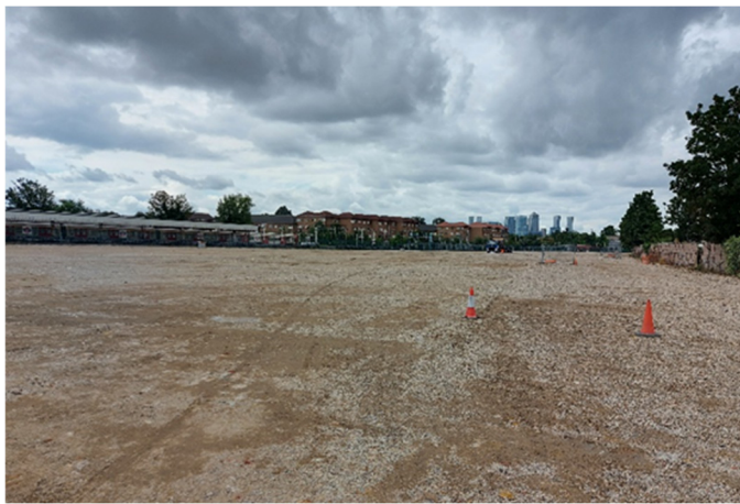
Figure 10: Photo showing the site following completion of works.
