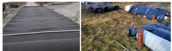
Figure 7: Rolled out RCM ® and OBB geo-composite. Figure 8: Cut and rolled up segments or panels.
