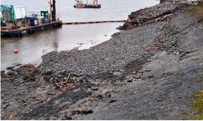
Figure 9: Area of filter stone placement.
