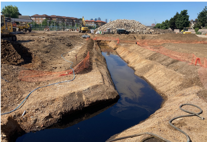
Figure 6: Recovery trench constructed in north eastern source area.
