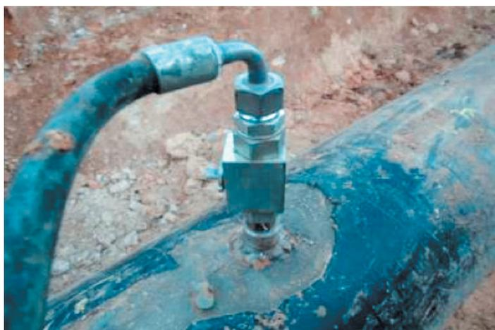
Left: an illegal tapping commonly includes a valve welded to the pipeline wall, and a length of flexible hose leading to a collection point which may include temporary storage facilities.
