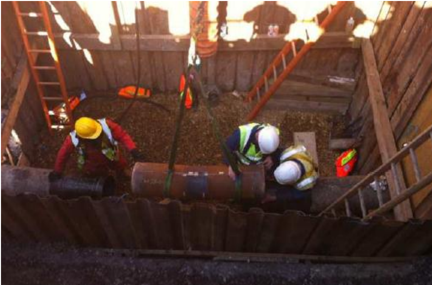
Installation of formed pup-piece
