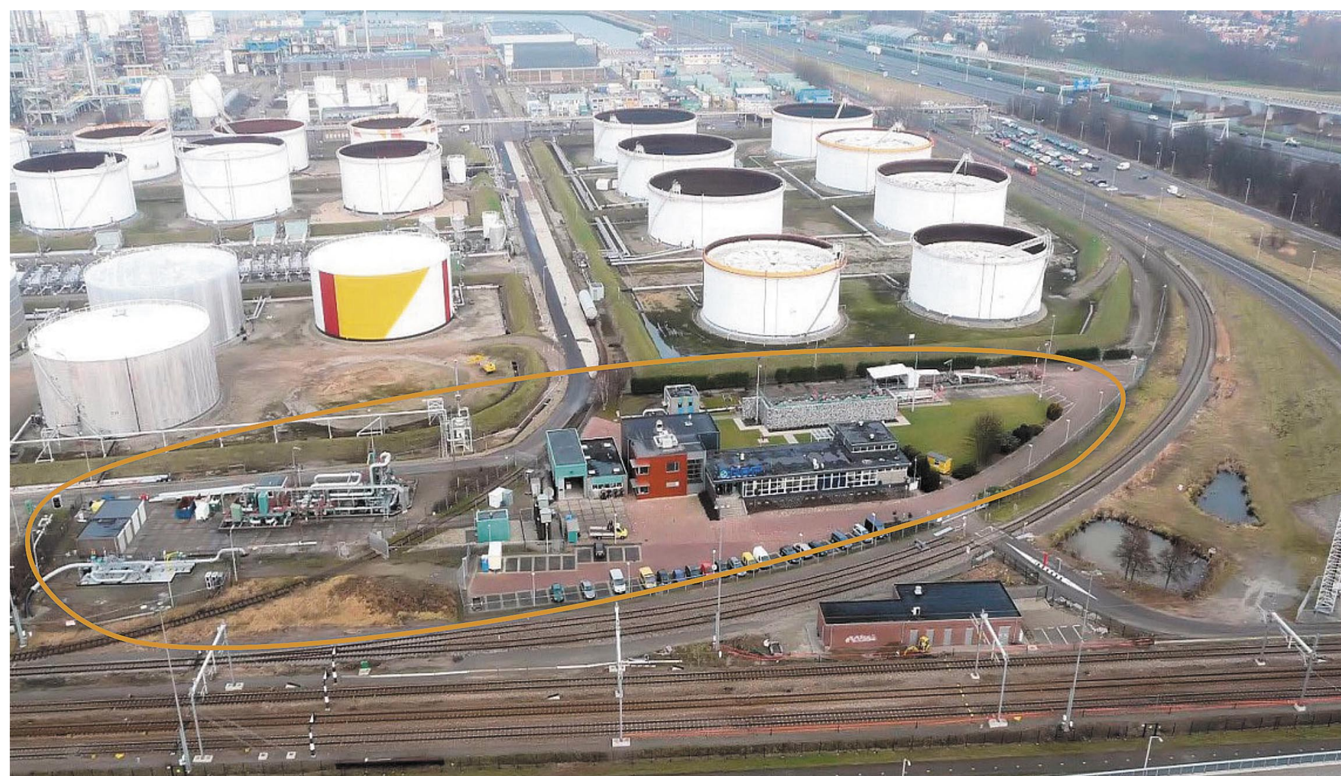
Pump Station Pernis
