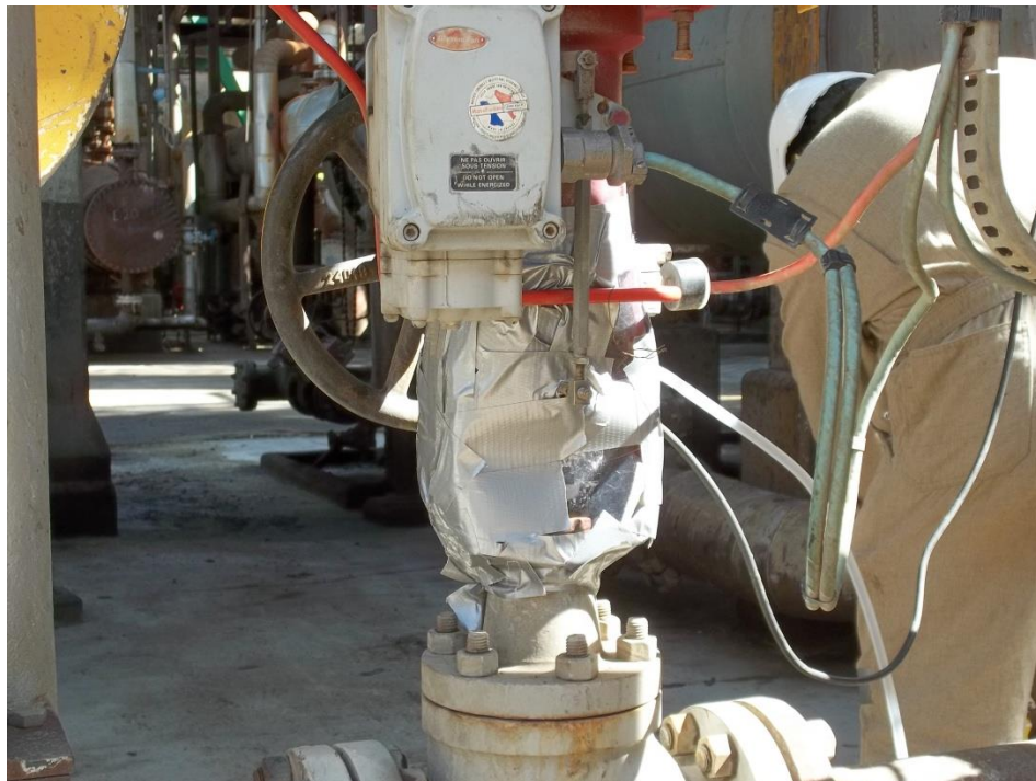
Figure 6 Image of vacuum bagging performed on a leaking control valve
