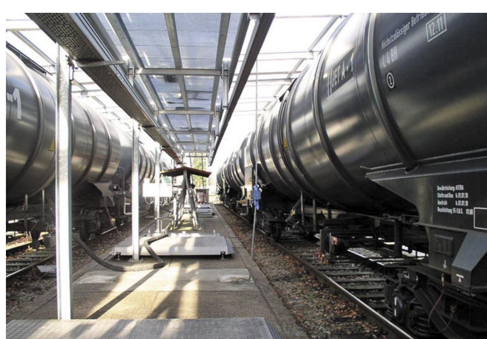
Rail loading station
