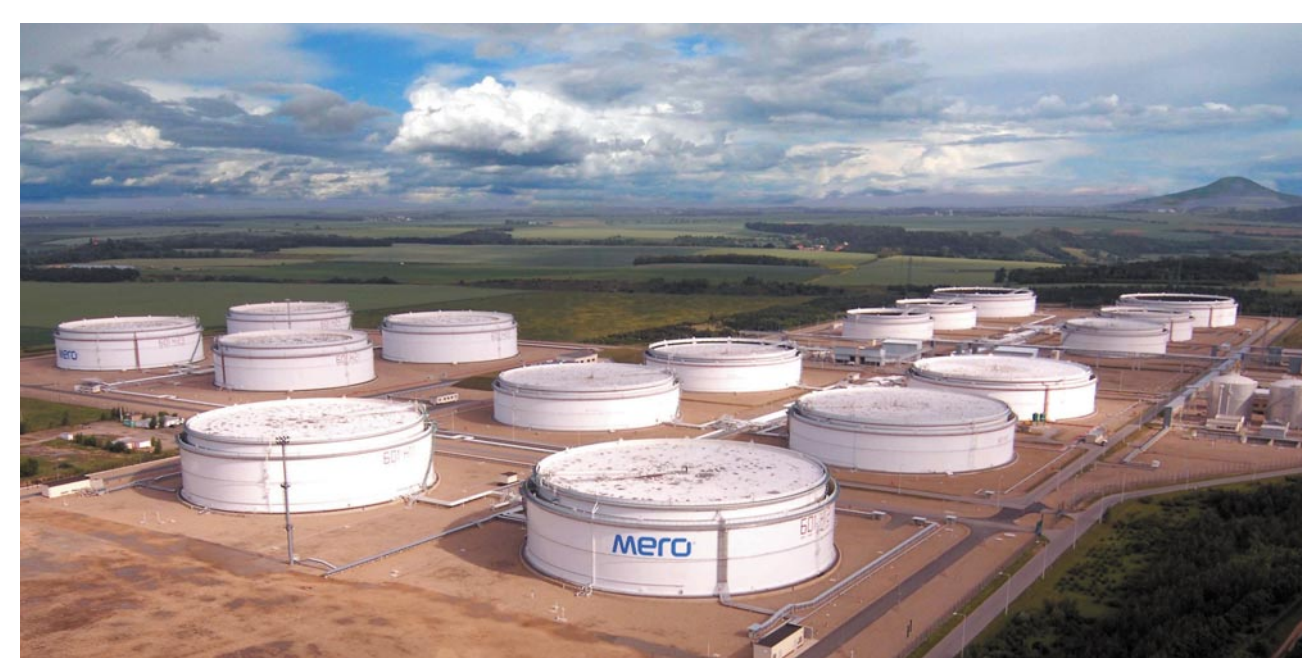
Central tank farm at Nelahozeves
