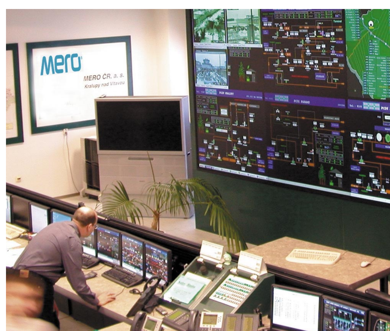
Control room at Nelahozeves
