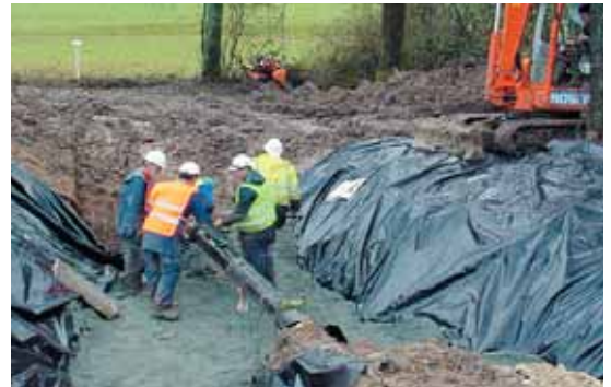
Repairing a damaged pipeline
