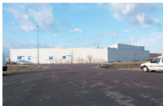
A typical blastproof control room
