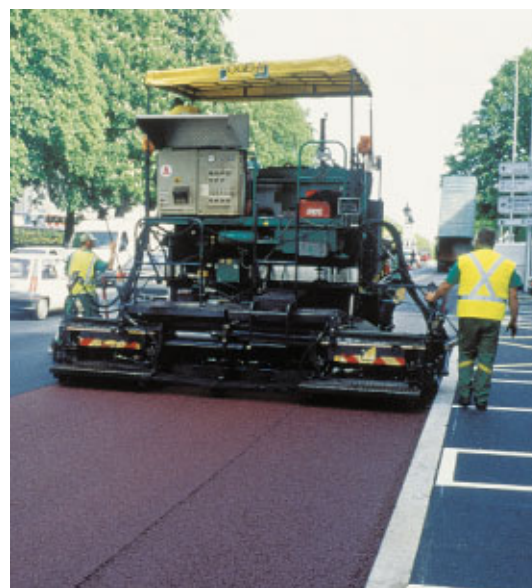
Asphalt road paving under way
