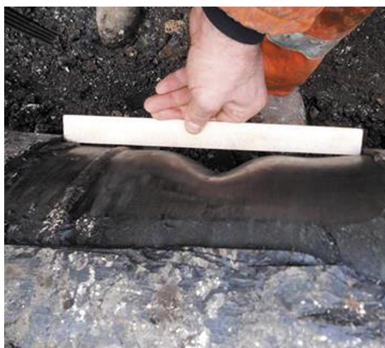
Pipeline dent—investigated and repaired
