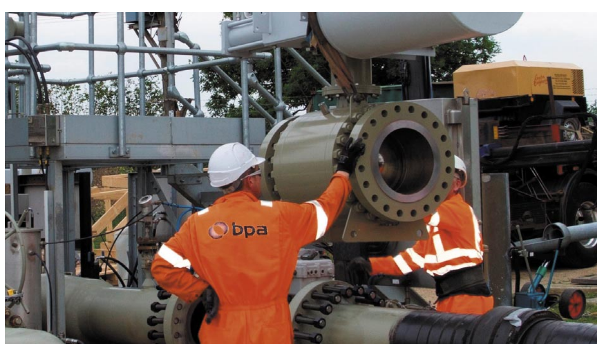
Engineering pipeline systems
