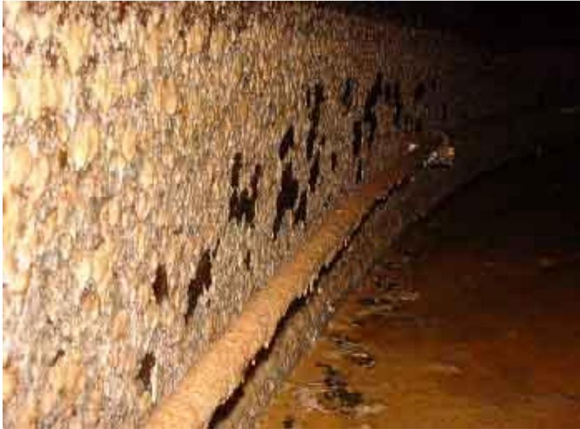
**Slimy deposits at wall and bottom of a B5 terminal tank**
